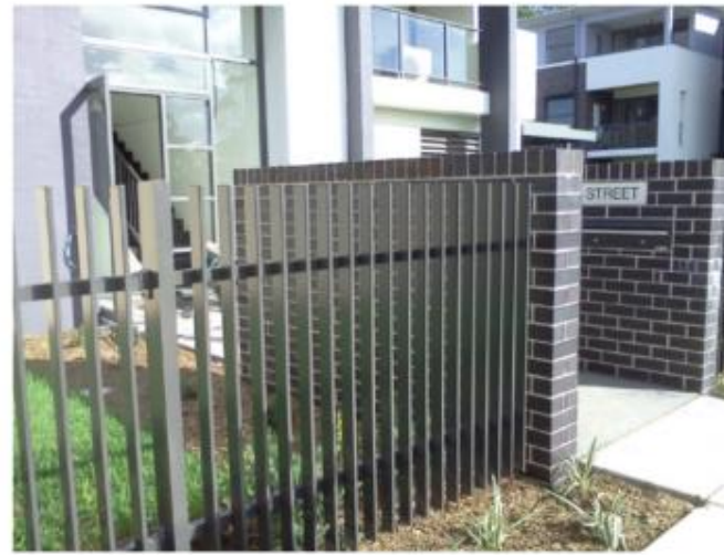
PROPOSED 1200mm HIGH VERTICAL PALISADE BOUNDARY FENCING & BRICK BLADE WALL WITH LETTERBOXES
