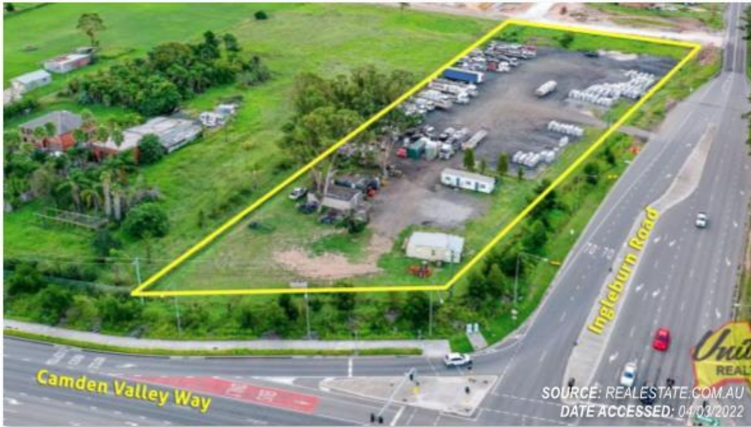
FIGURE 9: VIEW OF THE SITE TO THE WEST FROM CAMDEN VALLEY WAY INTERSECTION
