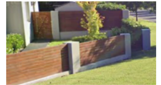
Sample masonry posts with timber infill and timber gate.
