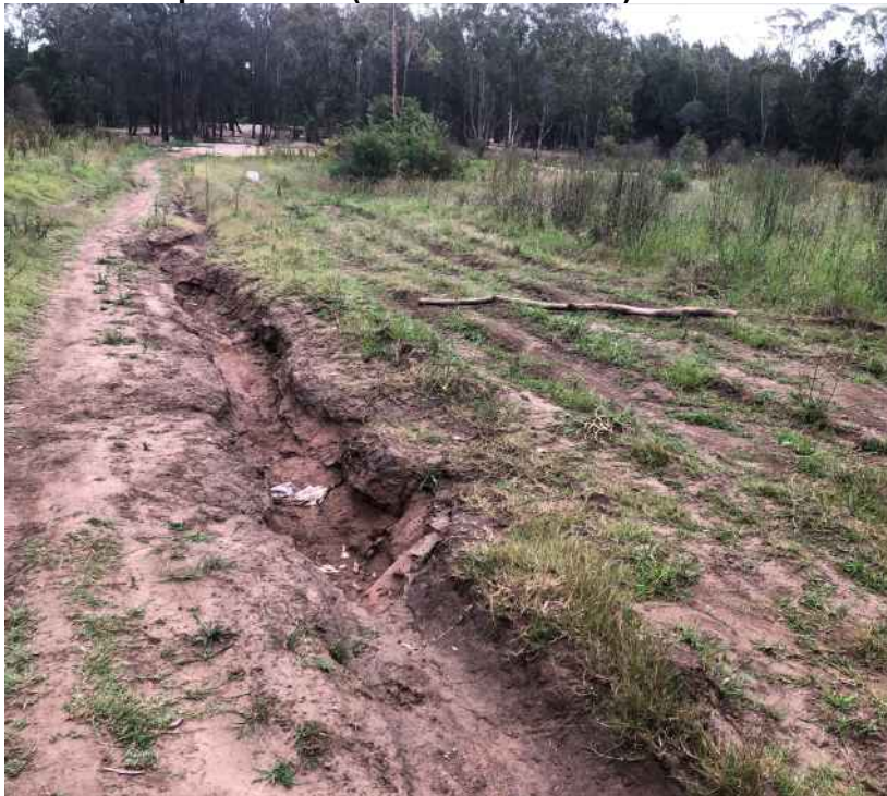
Image 10: Overland flow erosion gulley alongside vehicle access track looking towards Nepean River (1 December 2022)
