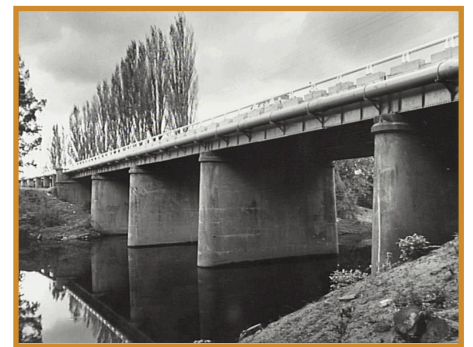
1976 - Cowpasture Bridge at time of official opening after repairs.
