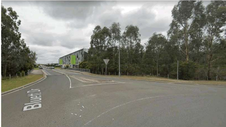
Figure 4 View towards site from southwest Source: GoogleMaps
