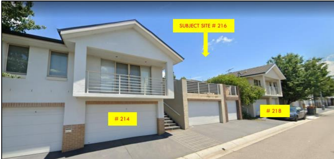
Figure 3: Subject site – View of site from Stipa Lane
