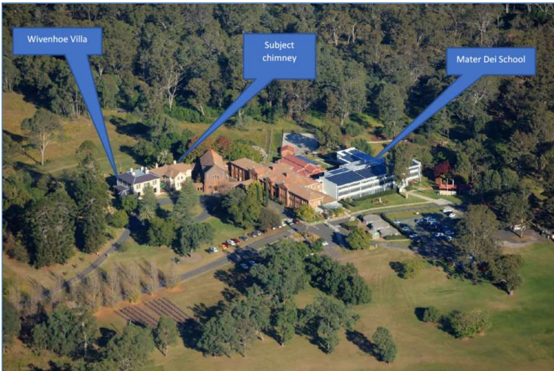
Figure 5: Specific aerial view of the site with the subject chimney for removal.
