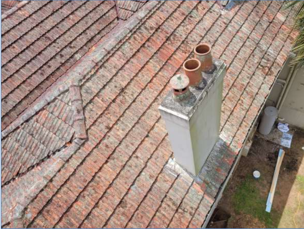
Figure 8: Subject chimney for demolition.
