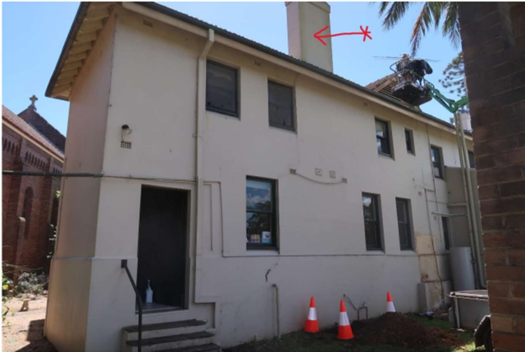
PHOTO 1: Chimney – south wall
