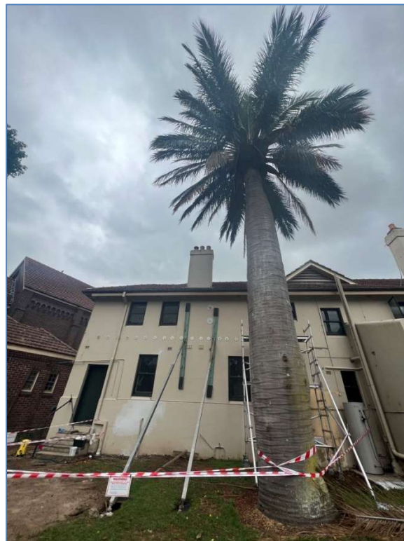
Figure 9: Current view of south western wall and subject chimney
