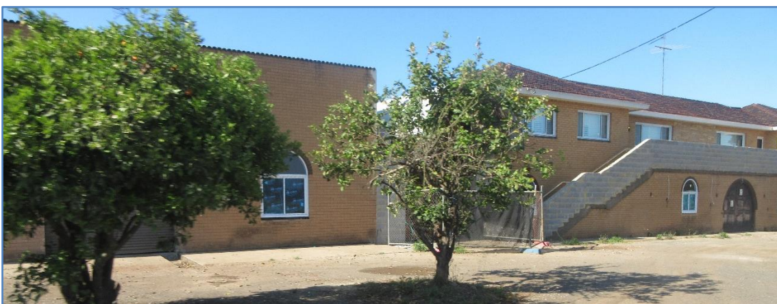
Figure 3 – Front elevation of the development site (as viewed from Cobbitty Road).
