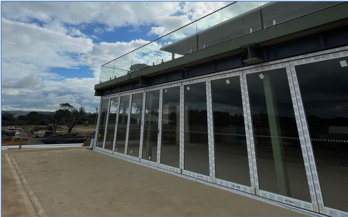
Figure 7 – Rear elevation of the main building with the unauthorised extension that is proposed to be used.
