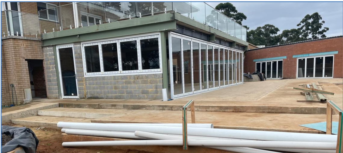
Figure 5 – Rear elevation of the main building with the unauthorised extension that is proposed to be used.
