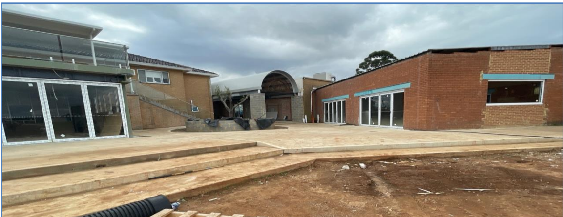
Figure 6 – Rear elevation of the main building and shed with the unauthorised extension that is proposed to be used.
