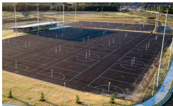
Wide view of the Narellan Sports Hub complex upon completion.
