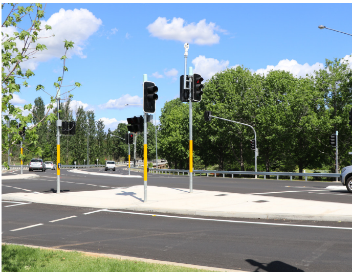
The upgraded Camden Valley Way and Macarthur Road intersection.
