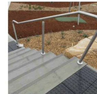
Stairs with handrail, tactile paving and nosing
