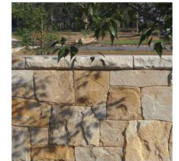
Sandstone Cladding to retaining wall
