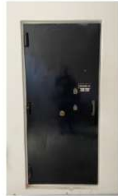
Figure 67: Safe to be retained.
