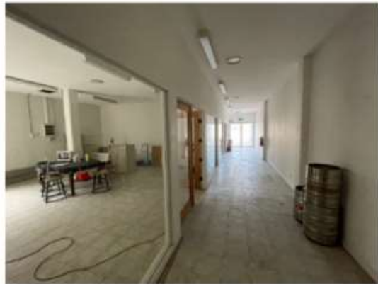
Figure 69: Recent walls proposed to be removed.
