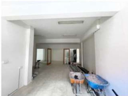
Figure 68: Rear of subject tenancy.
