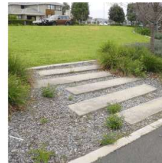
Precast concrete stepping stone
