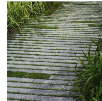
Paver arrangement next to mass planted area
