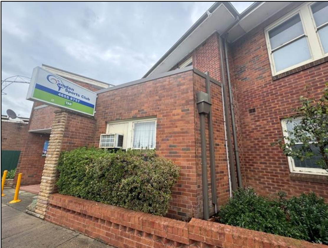
Figure 8: Site photo of existing external lobby area
