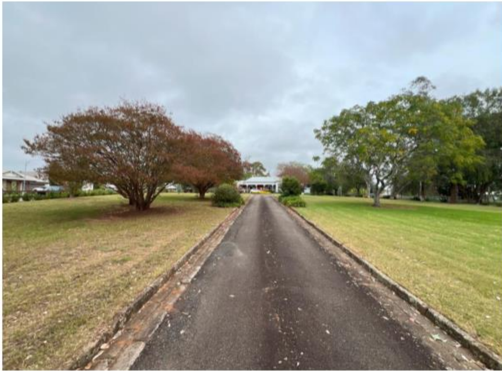
View from the bottom of the subject drive to the residence. Note sandstone guttering/kerbing.
