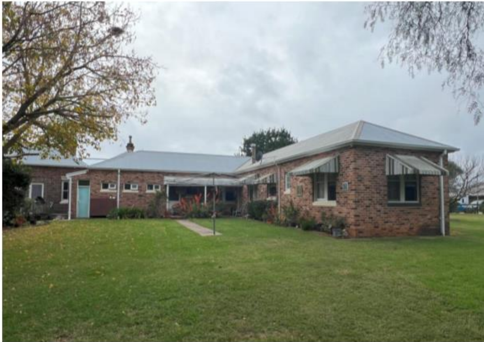
Rear elevation of the late 20 th -century rear addition, facing east. Main location of the proposed new works.
