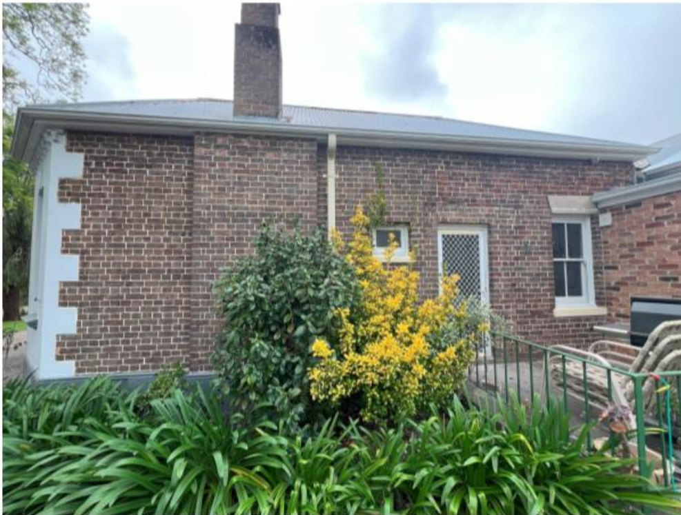
Rear (west) elevation of the early addition.
