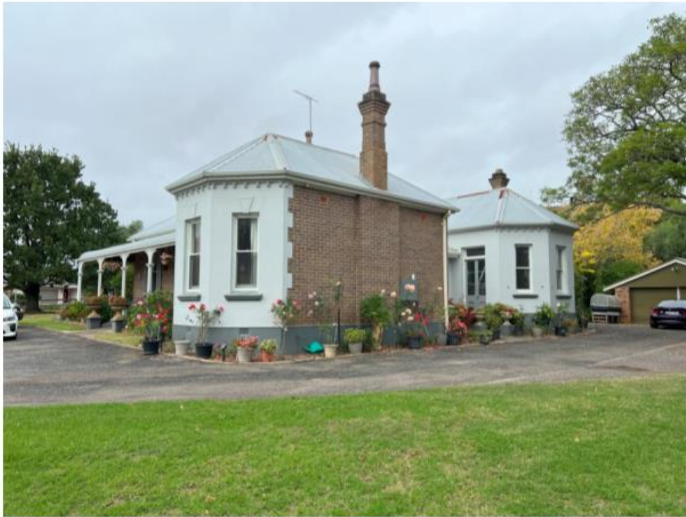
North elevation, facing west.
