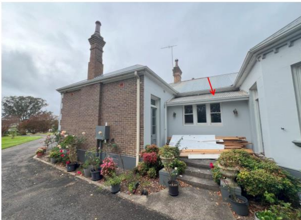
North elevation—showing the late 20 th century skillion-roofed 'link' (red arrow).
