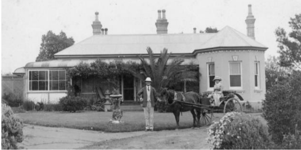
Mr and Mrs Fumer and their sulky, in front of Pammenter/Hillsyde's façade, early 1900s—post addition of the rendered wing (right). Note the enclosure of the return verandah's south-eastern corner, possibly an original feature, since lost. (Source: Camden Libraries, CH23305)
