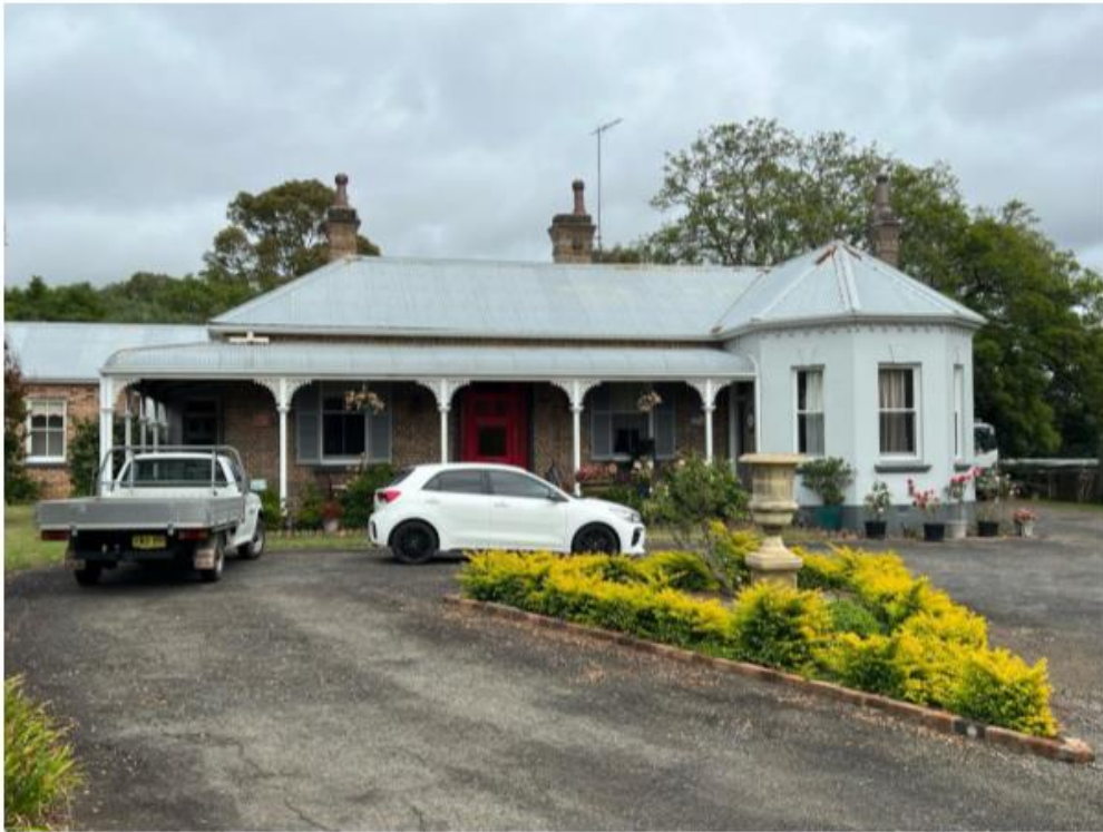
Façade, note the hybrid built form—original dwelling (symmetrical, brick, hipped) with rendered addition (probably Federation).
