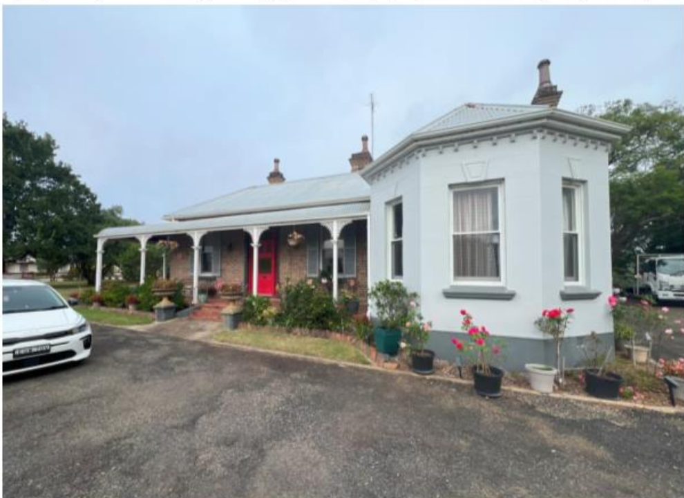
Close-up of the façade.
