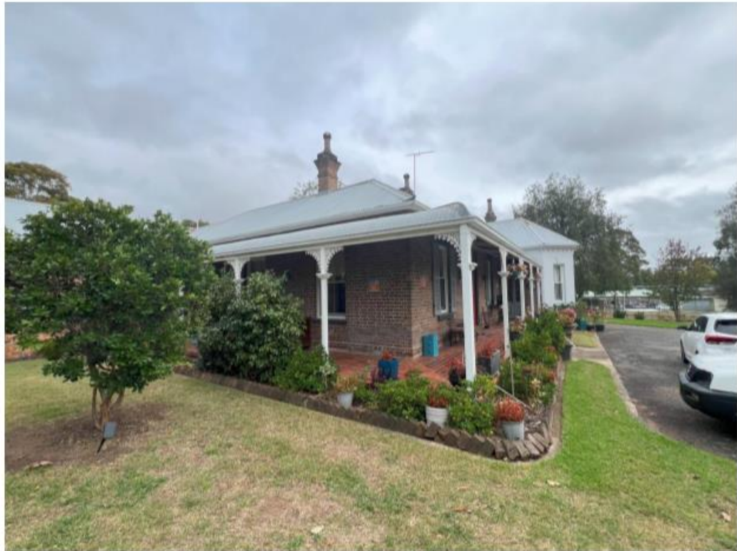
South-eastern corner of the subject residence.
