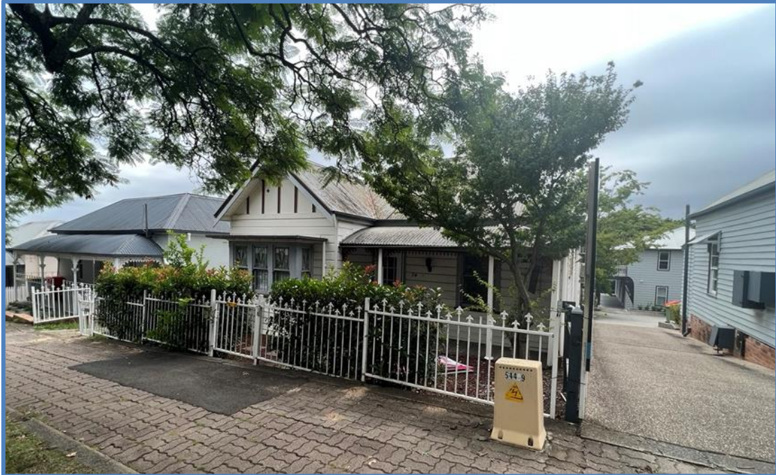
Figure 5: Site photo of the existing heritage cottage from John Street.
