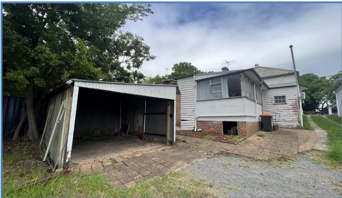
Figure 6: Site photo of the existing heritage cottage from the rear elevation.
