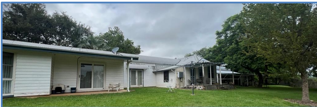
Figure 7: Existing single storey dwelling proposed to be demolished.
