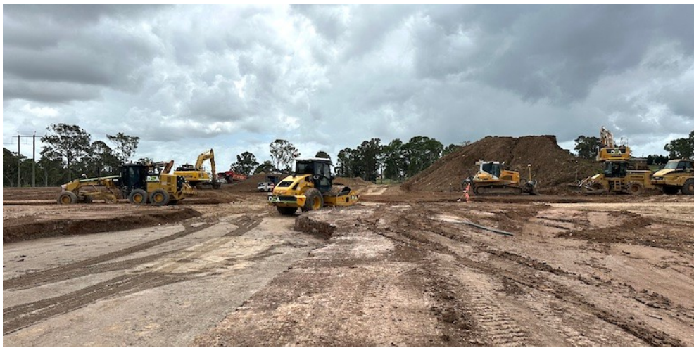
▲ Work under way on one of Castle Group's Camden sites.
