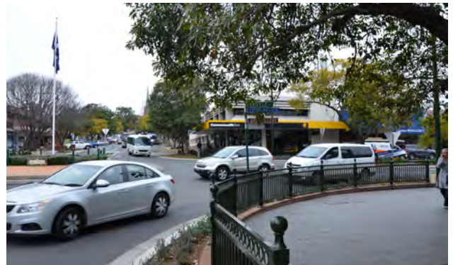
Intersection of Argyle and John Street upgrades
